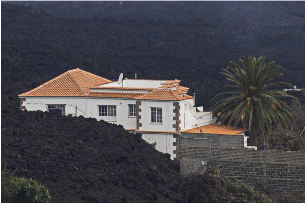
FIG. 13 – (Upper) Lava destroyed more than 2000 buildings. (Lower) This house was spared destruction but was left surrounded by high lava walls.
